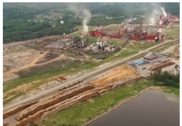
Vyborgskaya Cellulose pellet plant, Leningrad Oblast, Russia. GPS: 60.5472053, 28.6727205. Still image from "Bioenergy: The Ugly Truth" 38
